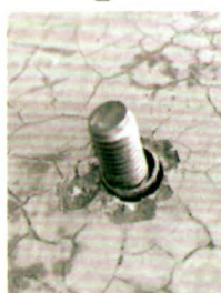
3. Place the expansion screw into the hole.
