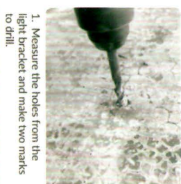
2. Drill 2 holes with an M10 drill bit on the surface according to the two marks.
