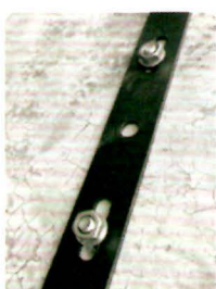
1. Measure the holes from the light bracket and make two marks to drill.
